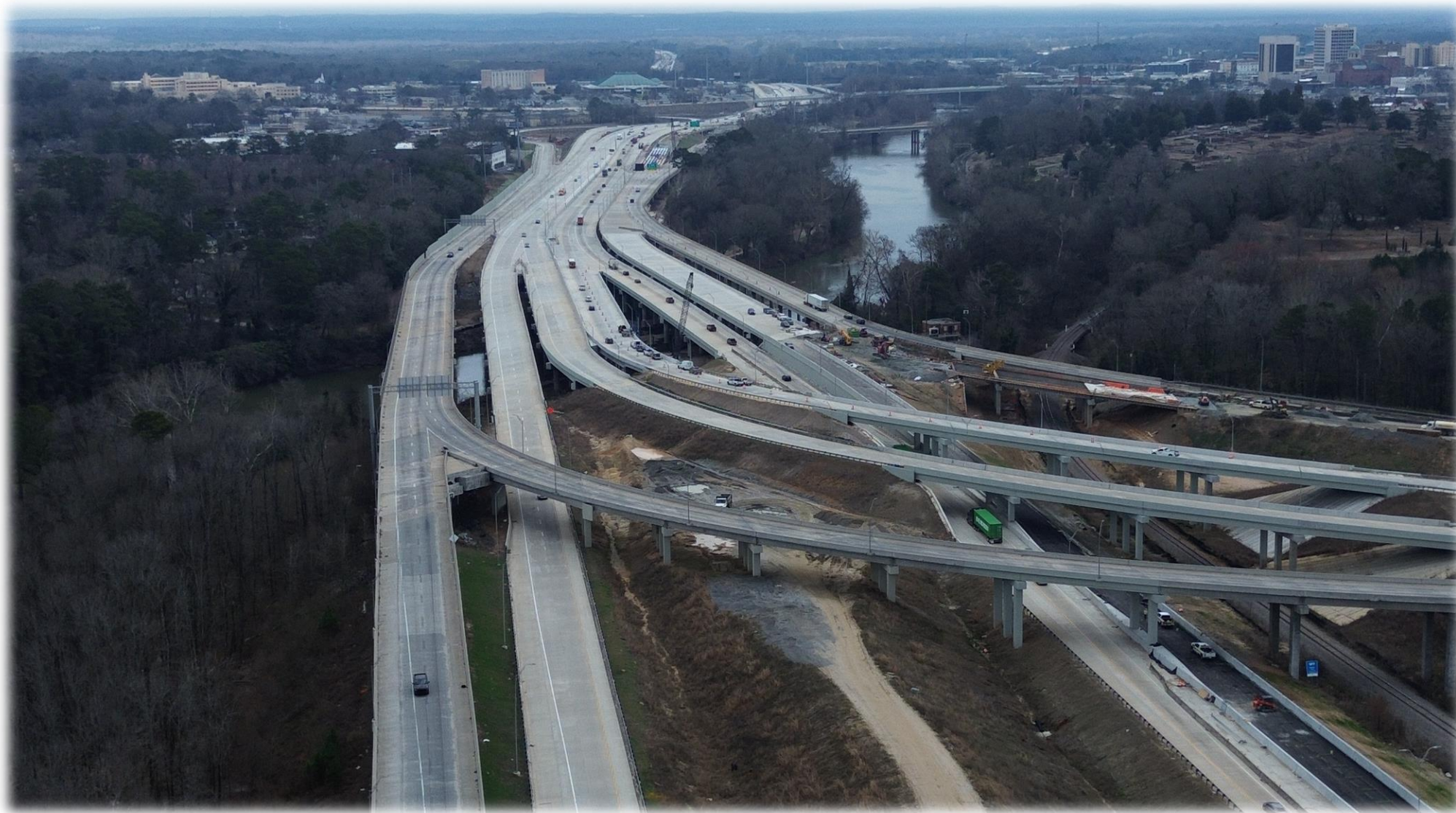
I-16, I-75 interchange facing east
