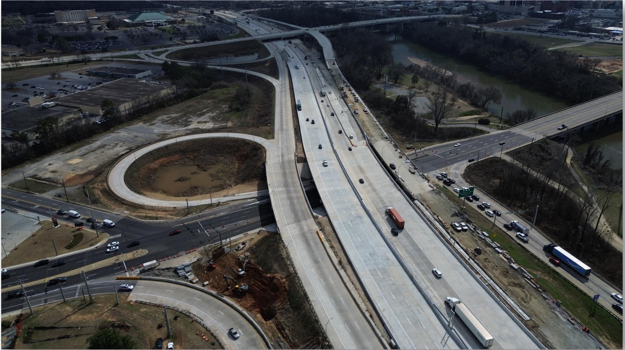
Spring Street interchange
