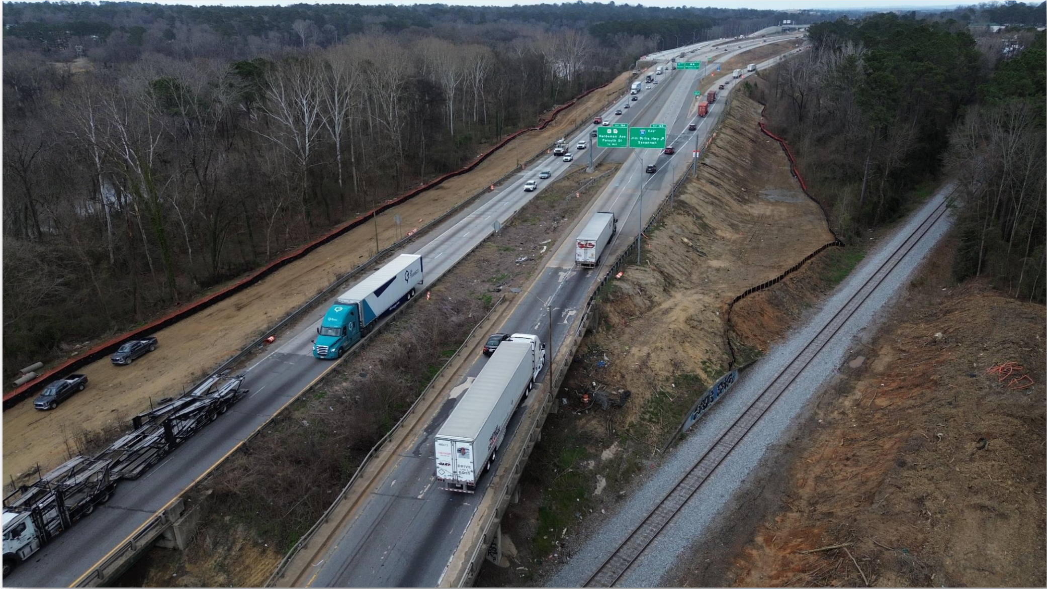
Phase 6 looking southeast
